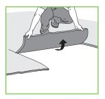
If you are going to carry out the installation a room with flooring already installed, remove all unsuitable coverings (carpet, felt, old floating floors, CV coverings, etc.) before installation. Coverings such as hard PVC, linoleum or tiles do not need to be removed if they meet the conditions mentioned in the previous paragraph. When installing on a wooden floor, ensure its stability, screw in loose parts and lay a levelling layer if necessary. The subfloor must not be flexible
